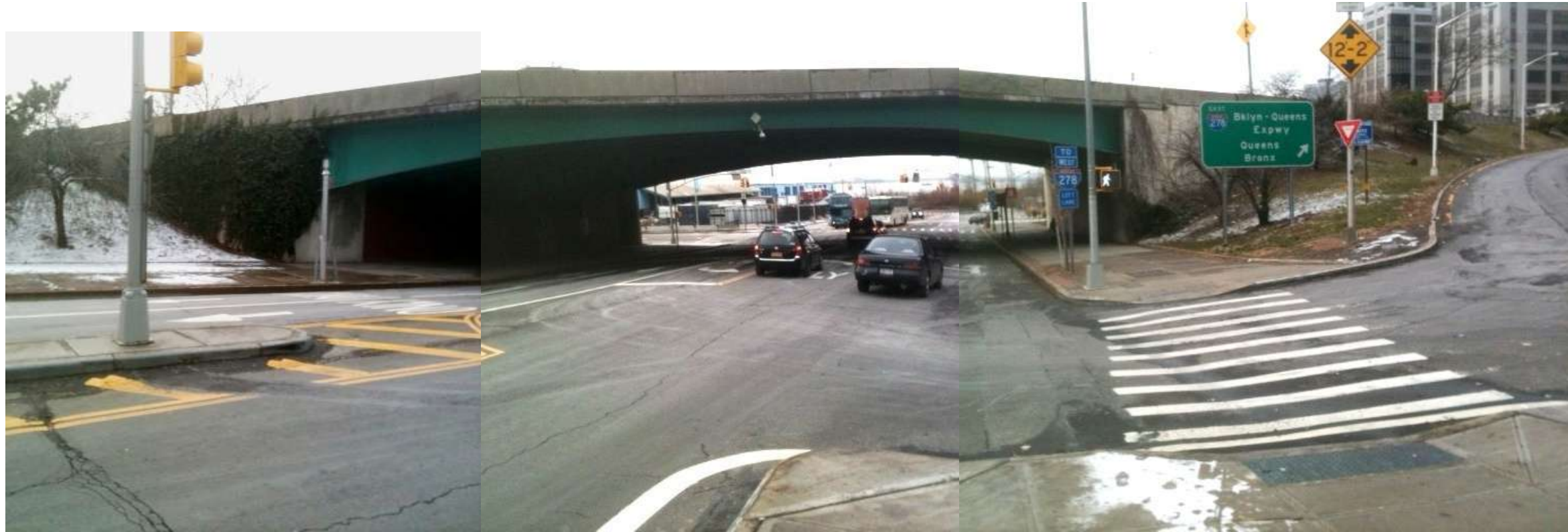
East Elevation BQE Underpass / Atlantic Avenue
