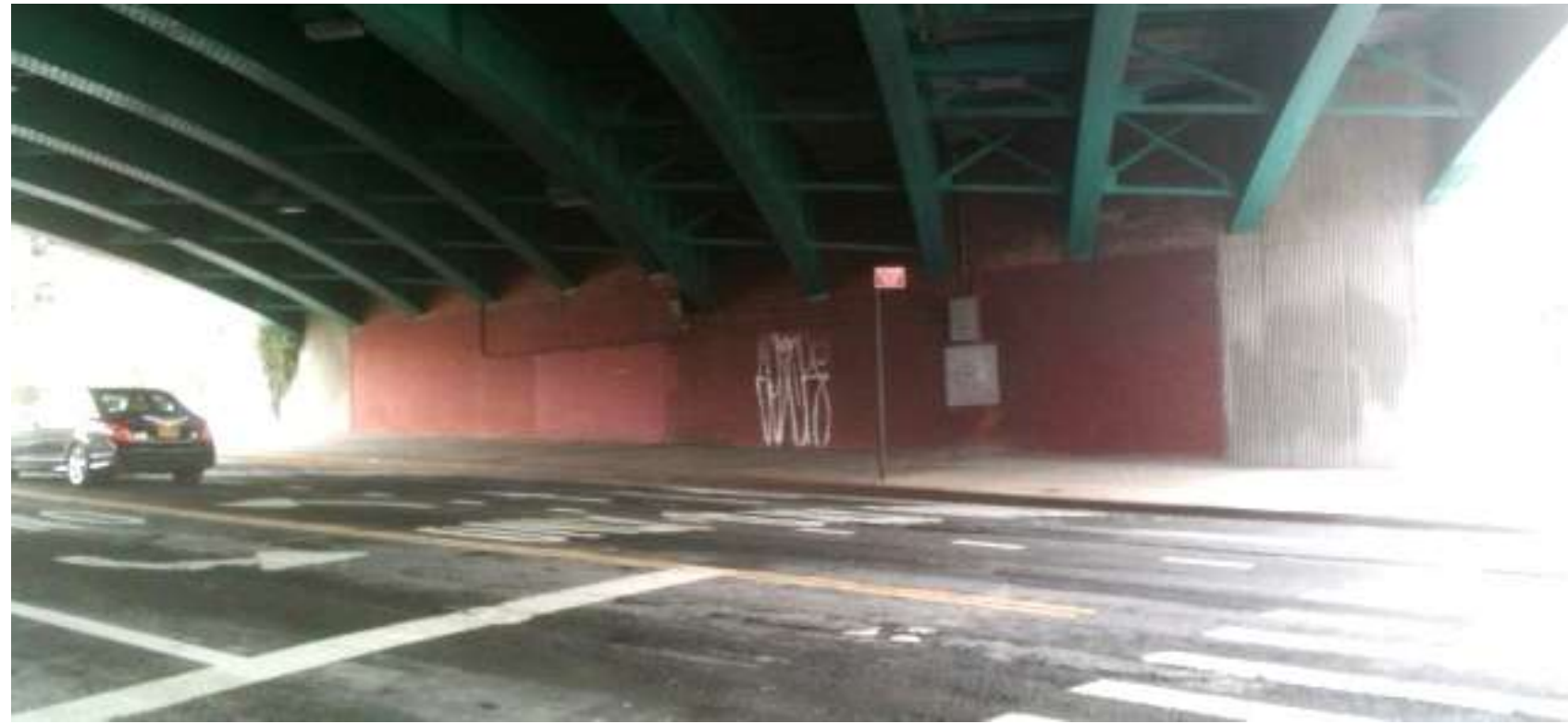
BQE Underpass / Atlantic Avenue – South Elevation
