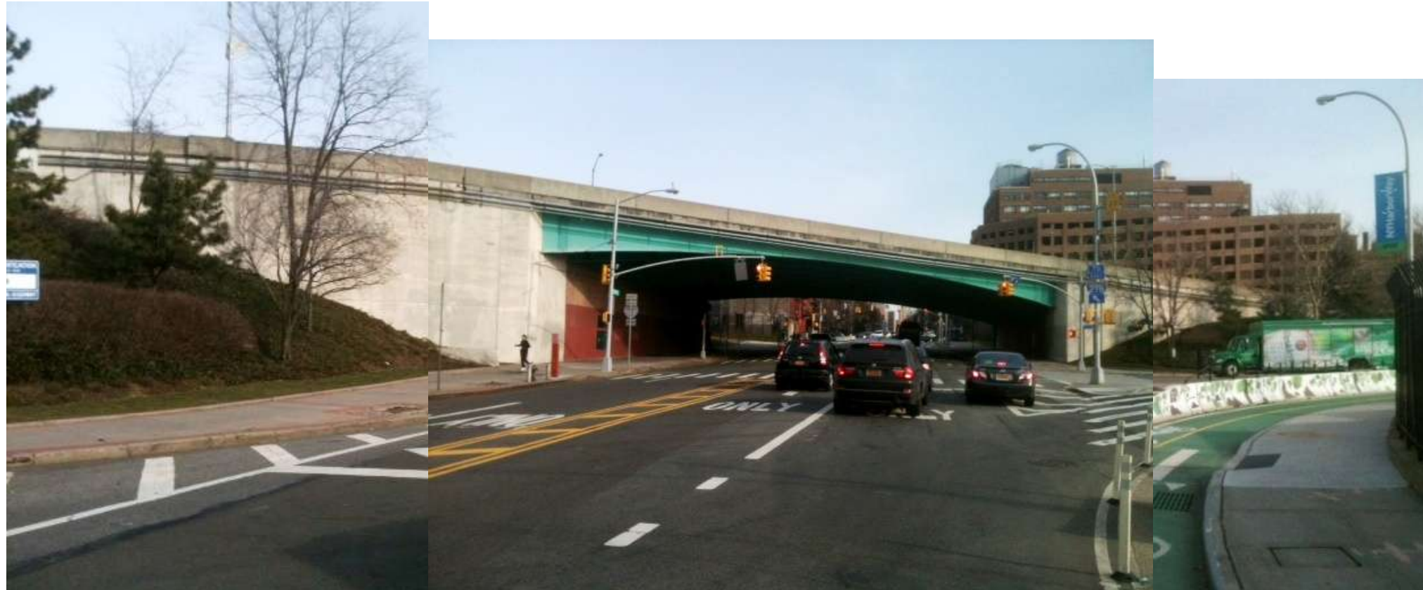
West Elevation BQE Underpass / Atlantic Avenue
