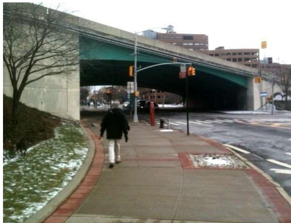
Furman Street into Atlantic Avenue - West of BQE Underpass
